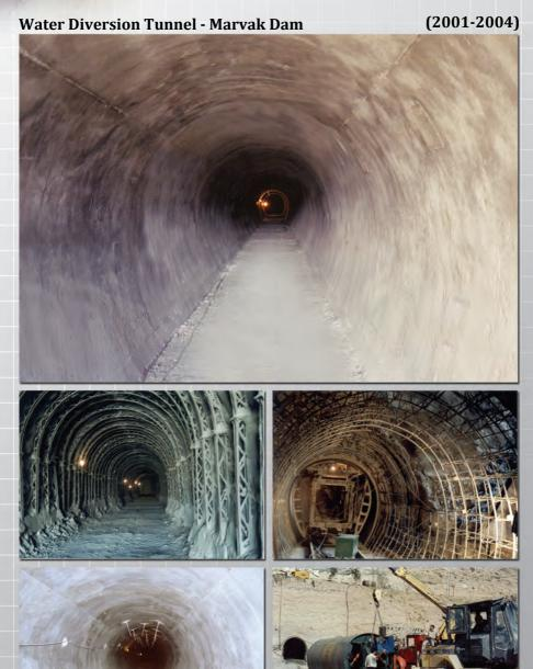
Including implemeting and excavation and lining of the two Tunnel, each 500 meter long and two vertical and one angled shaft (total length:120 meter) and their subordinate structures in beginning along and at the end of the part and also Pre-Constructing the camp and landscaping of the camp.
